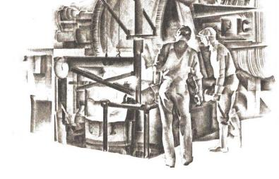
Ordinary cast-iron, as you may know, is produced by melting blocks of iron in a furnace-like structure called a cupola. The molten metal is then poured into molds and allowed to harden.
